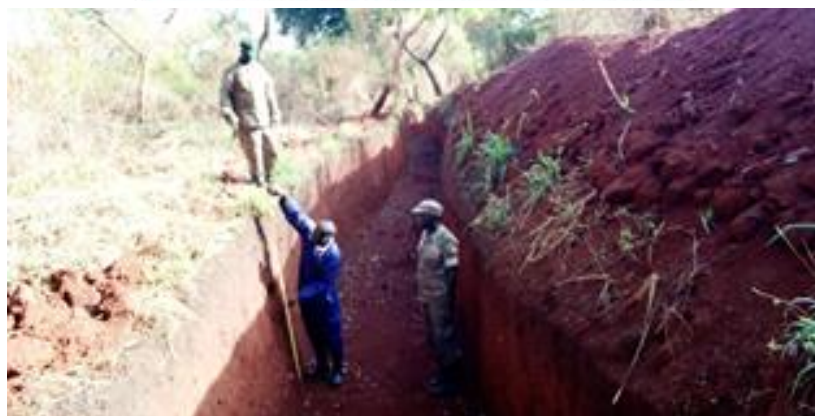
WCS Staff Measuring the dug trench with UWA ranger
